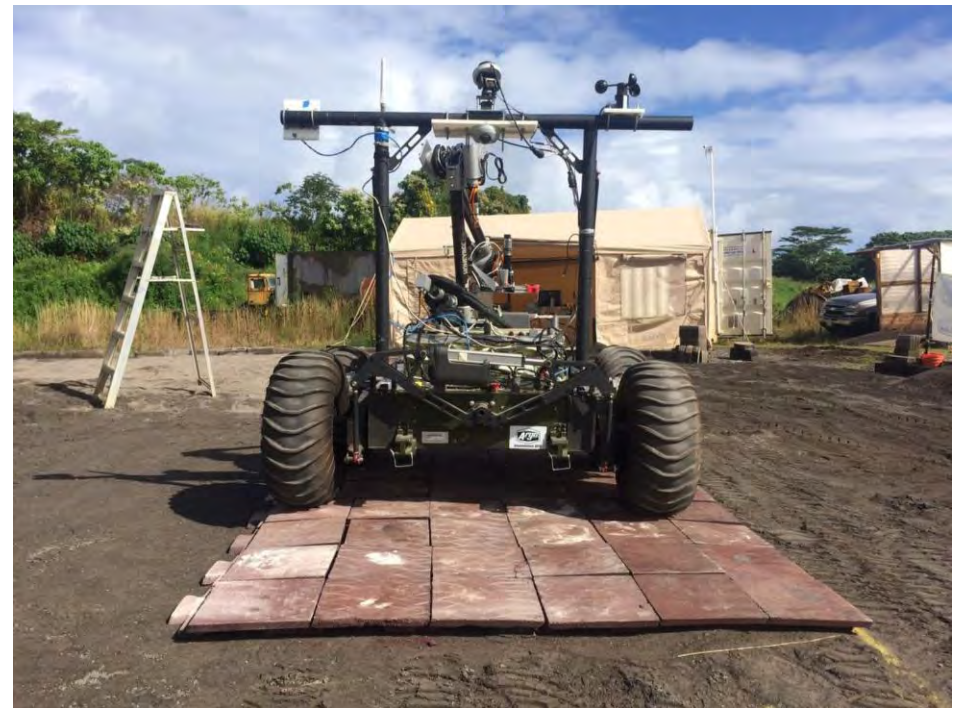
A rover built a prototype launch-and-landing pad on Hawaii's Big Island in late 2015. Credit: PISCES
